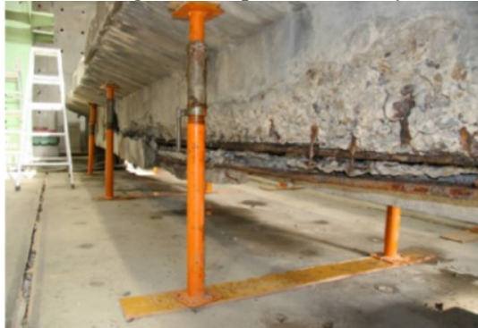
Figure 4: The validation beam from Nougawa bridge [15]
